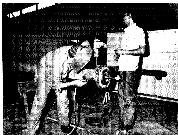
Figure 5. Welding Inconel-600 stub ends to the HK-40 catalyst tubes. Root run is being welded by the “tig” process with argon purge.
